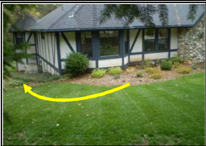
Positive grading directs water around house.
