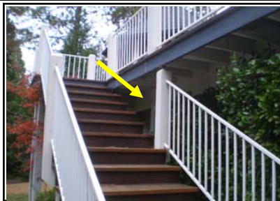
Missing railing noted on rear deck steps - hazard.
