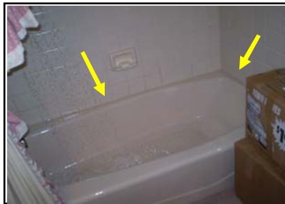
Recommend keeping seams & edges sealed.
