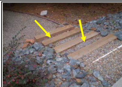
Uneven step surfaces noted. Hand rail recommended.
