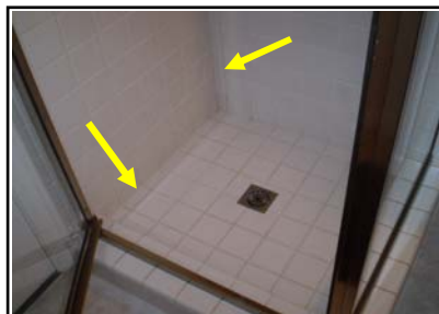
Recommend keeping shower seams & edges sealed.
