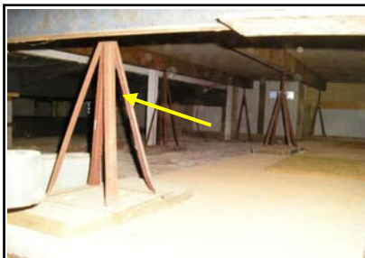
Steel jack piers noted under decking.
