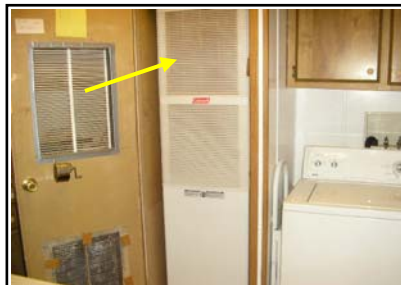
Furnace - return air filter located behind top panel.
