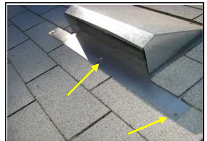
Caulking is recommended on exposed nail heads.
