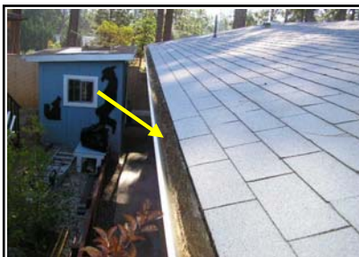
Debris noted in gutters.
