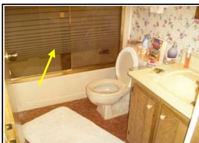
Bathroom # 2 - safety glass recommended for shower doors.
