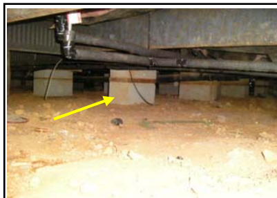
House supports are concrete block on wood bases.
