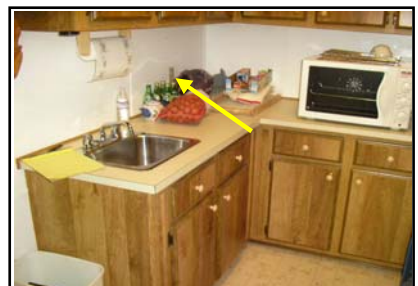
Laundry sink outlet not GFCI protected.
