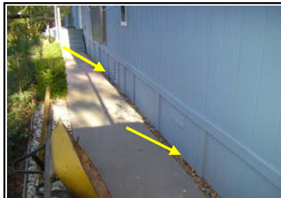
Negative grade noted along right side of unit.
