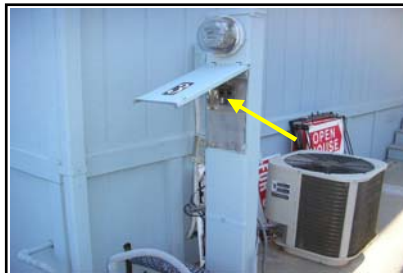
Main electrical disconnect.
